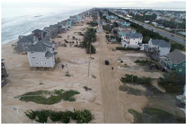
Avon Hot Spot is south of Rodanthe and north of Buxton. During storm events the ocean washes onto NC-12 because dunes have eroded leaving no real defense against over wash. Unfortunately, there are no viable outlets to allow the water on NC-12 to recede, so water stands on NC-12 for several days.
